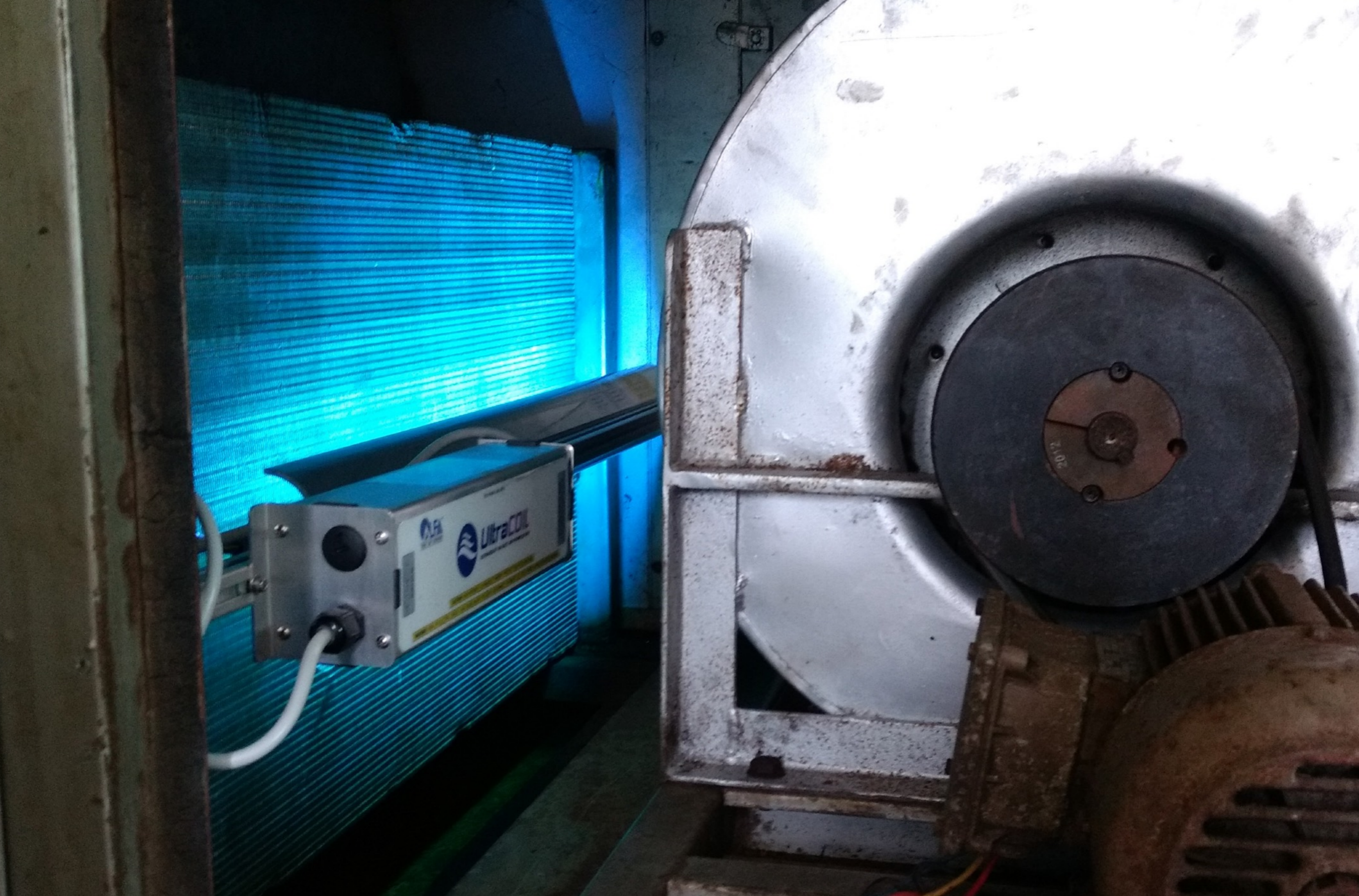
STANDARD INSTALLATION IN A LOW CAPACITY AHU
